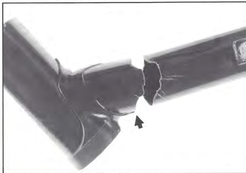
Figure 1: This fractured frame tube was weakened and may have failed from sand blasting.
